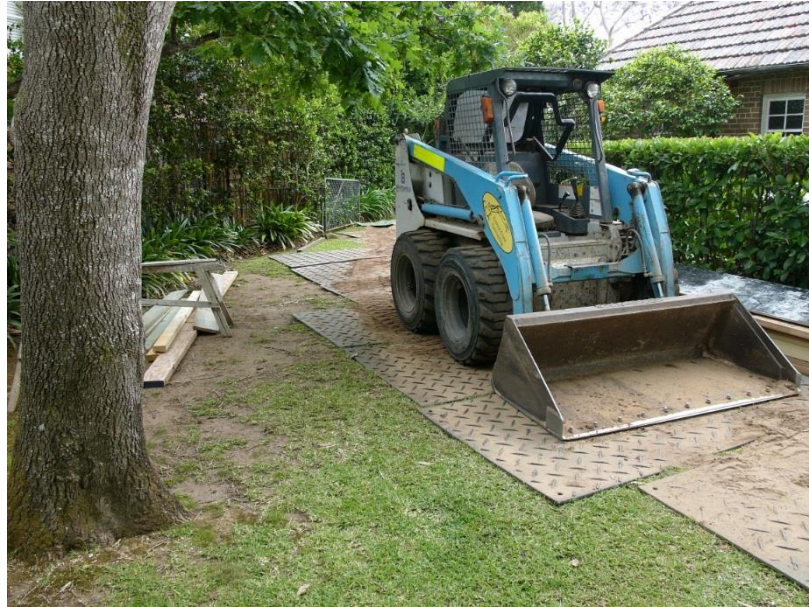
Figure 4 – Showing typical detail for truck mats.
